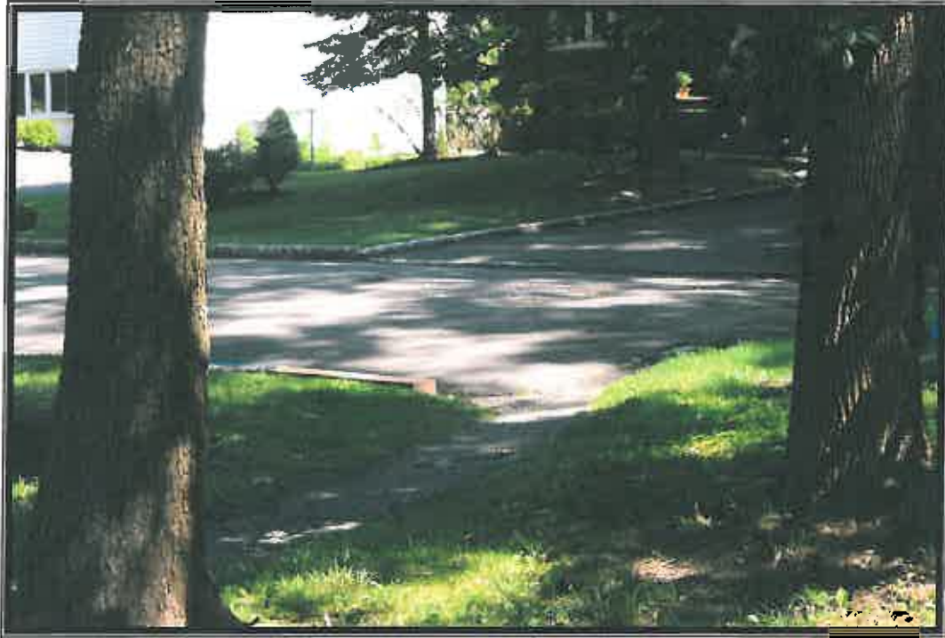
Figure 2 Showing Stormwater Catch basin at end of Cornell Street
