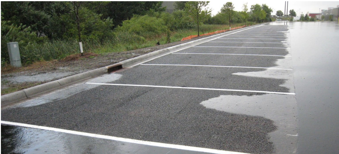
Example of permeable pavement (Source: Potomac Conservancy)
